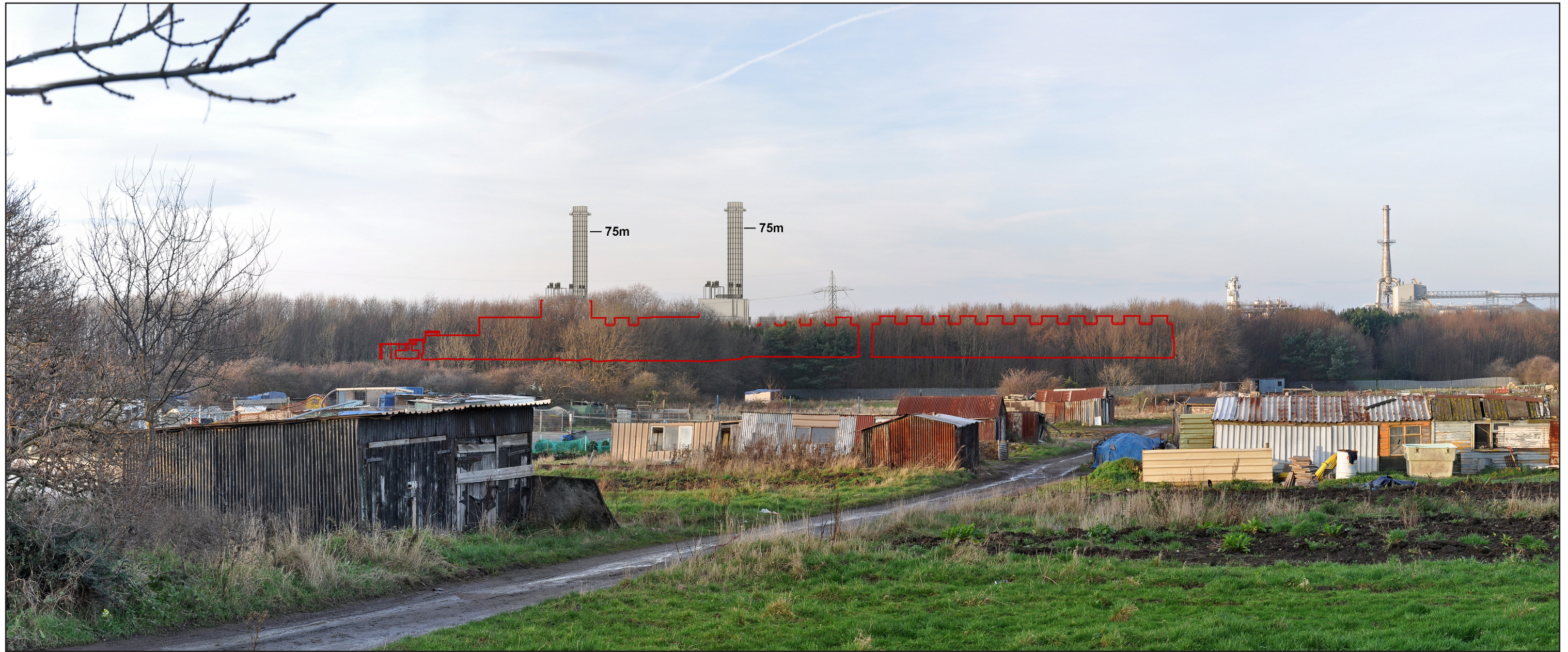
Wireline with outline of hidden plant in red
